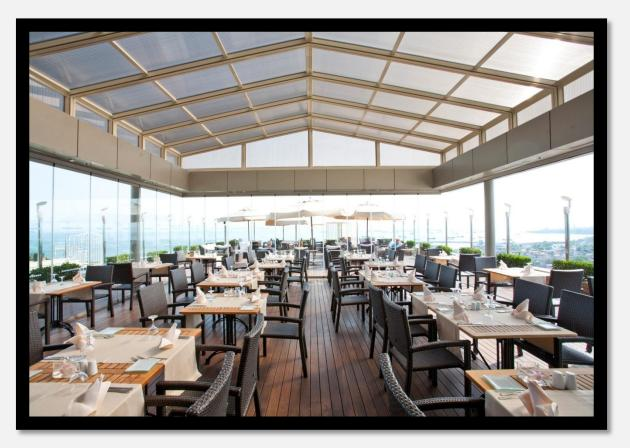
The Telescopic System consists of a fixed and a modular structure. Movable modules are retracted into the fixed module manually or with the help of an engine.
